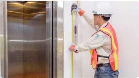
New Lift Installation
